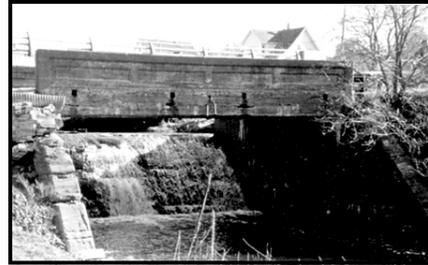
Built along with the first bridge in 1923, the Humphreys Mill dam was used for providing power to the Humphreys textile Mills. The present dam is not the first dam built on the site, since activities associated with the Humphreys textile and wood mill can be traced back as early as the 1820 s.
